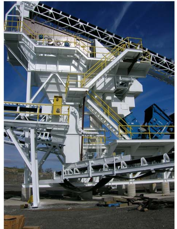
SCREEN AND CRUSHER SUPPORT STRUCTURE
