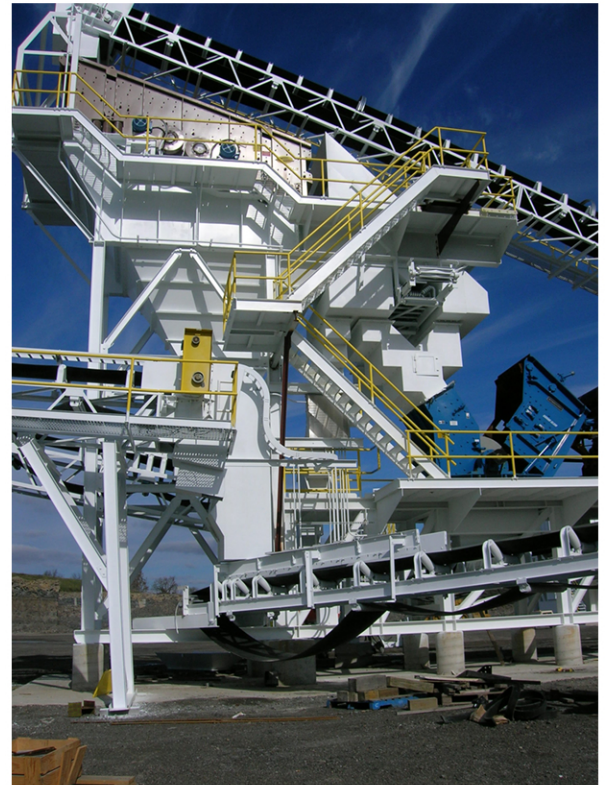
SCREEN AND CRUSHER SUPPORT STRUCTURE
