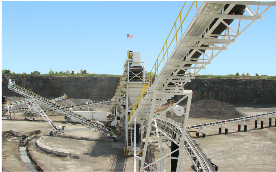
CONVEYORS IN AGGREGATE FACILITY
